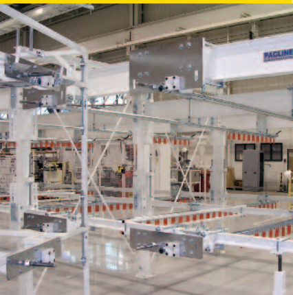
Cart and structure connecting
