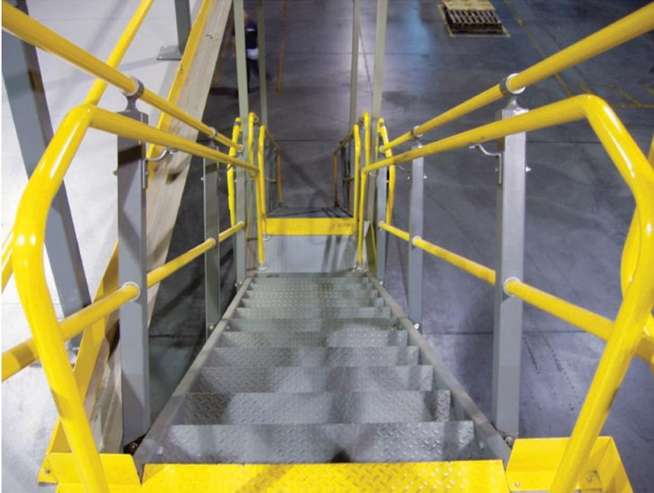
*Wildeck's Knock-Down Stair system was easily installed allowing REHAU employees to access the upper level. A landing was added to the long stair run to ensure employee safety.*
