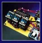
Heavy Duty Controls Designed for a clean, open layout to maximize performance and ease of maintenance. Contactors are oversized for increased life. Panels are housed in a dust resistant compartment designed for easy access and serviceability. (Actual hoist control may not be exactly as shown)
