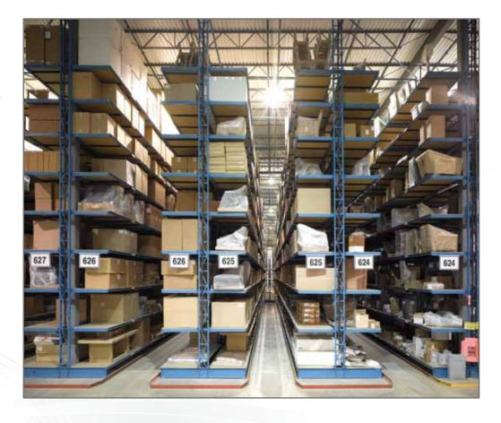
KONSTANT® engineers designed the very first Rack Supported Building. The strength of our rack easily supports the roof and walls of this freezer, creating an economical storage solution.
