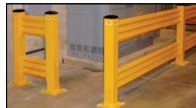
Guarding Electrical Panels
