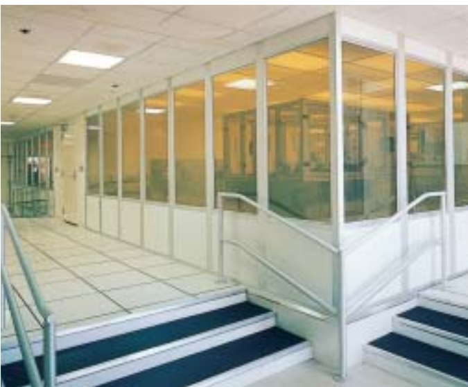
Cleanroom with raised floors in an R & D facility.
