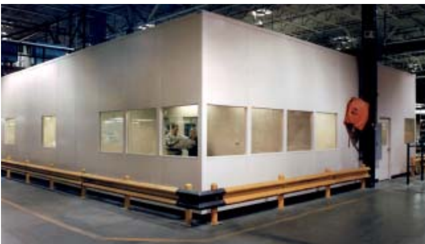
Office complex with protective guard rail.
