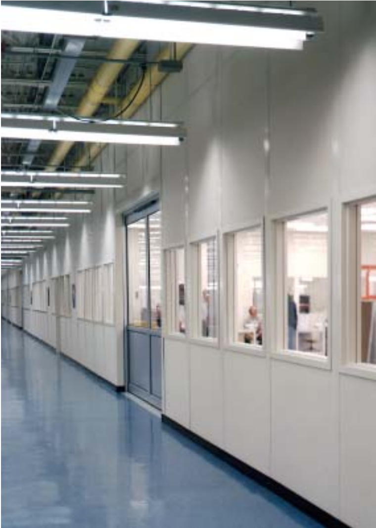
Environmentally-controlled enclosure for manufacture of intricate electronic components. Electronic sliding door.
