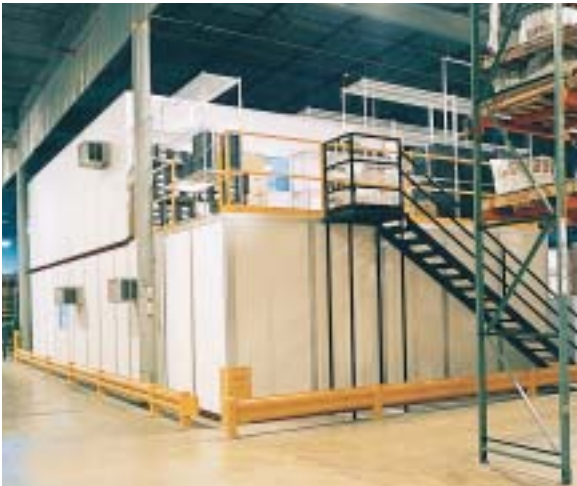
2-Story office complex with roof top storage area.
