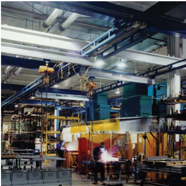
Aluminum Work Station Bridge Cranes
